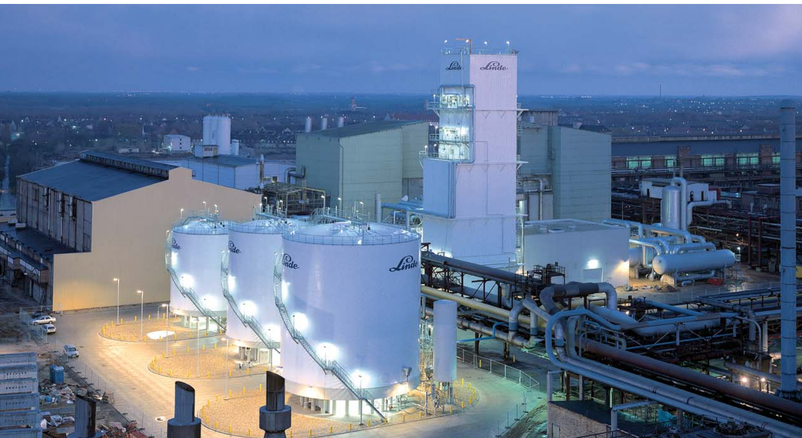
Air separation plant in Leuna, Germany
