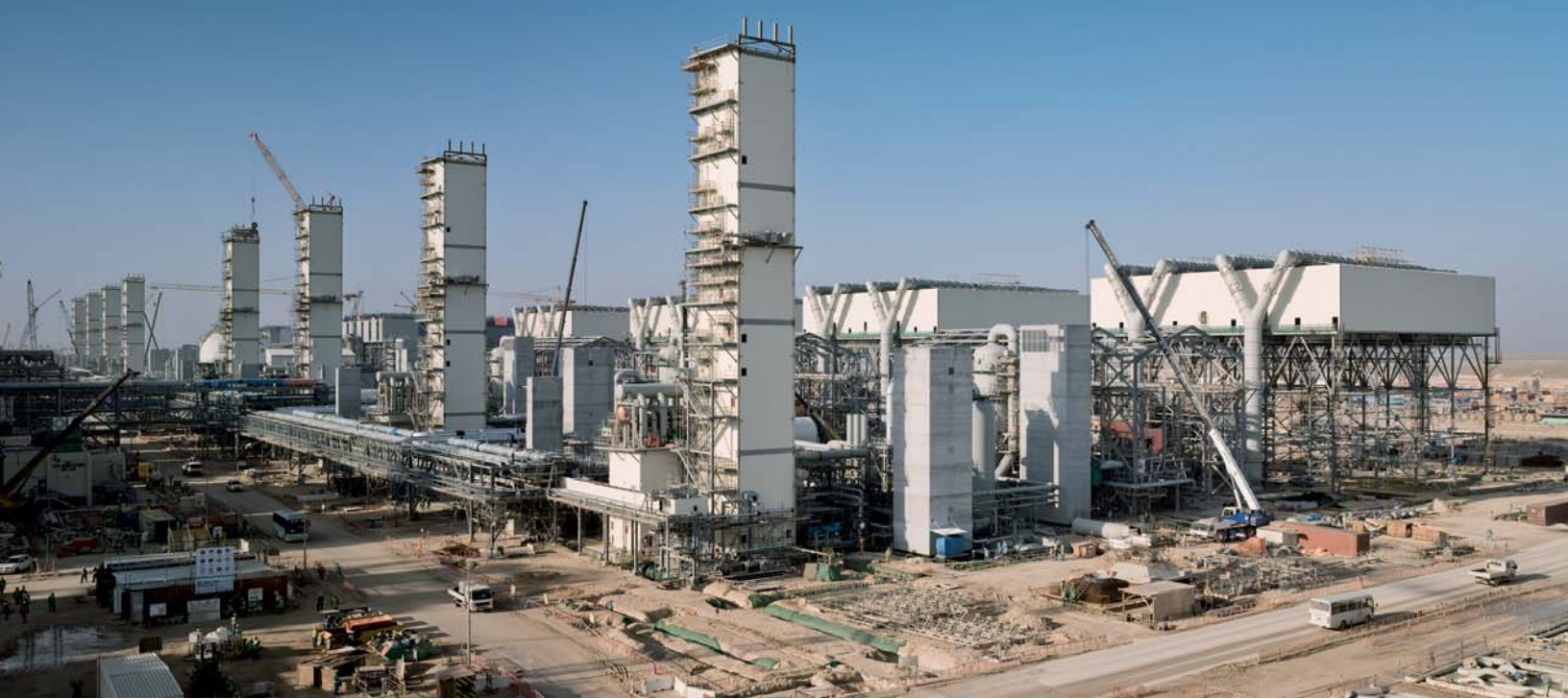
Shell "Pearl" GTL project under construction
