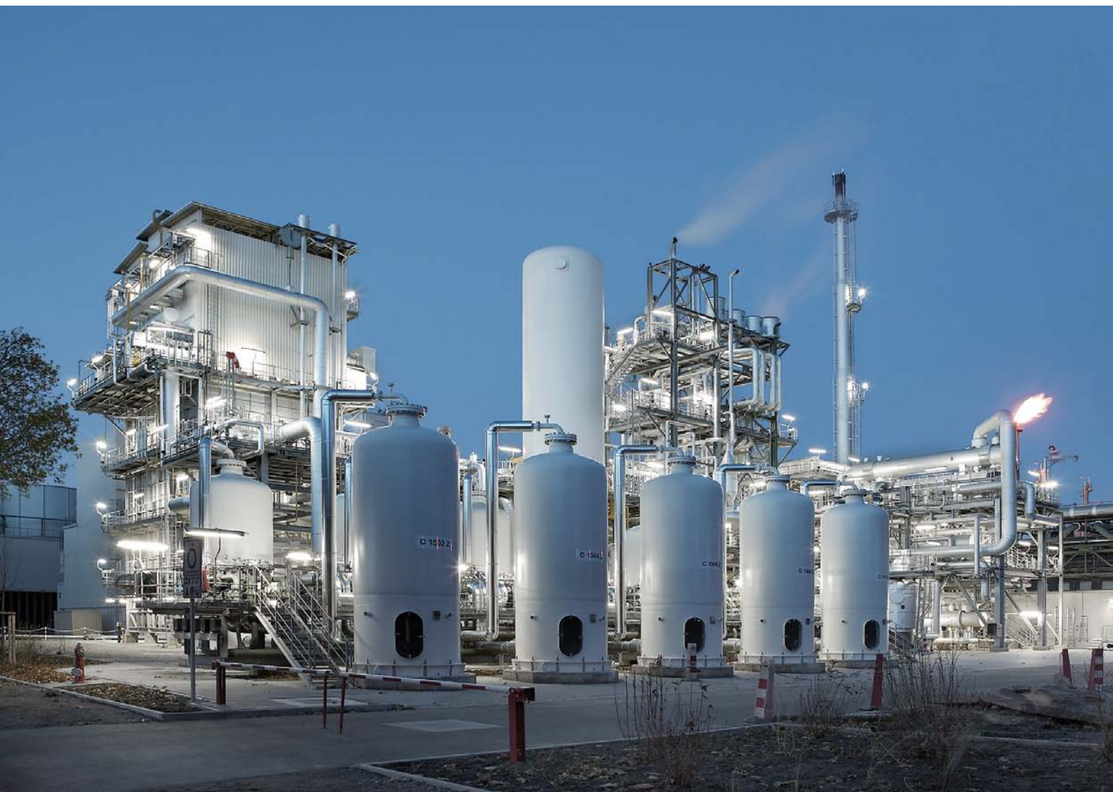
Hydrogen plant in Germany
