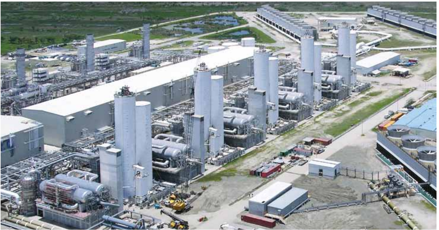
EOR plant in Cantarell
