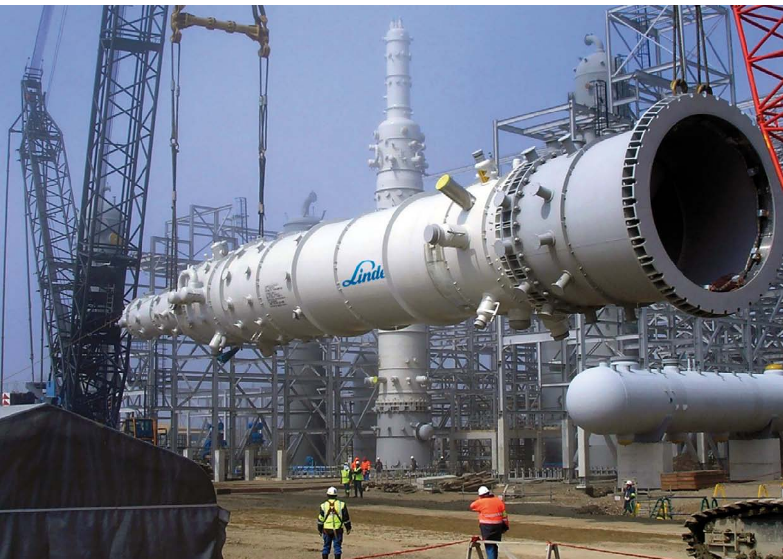
Complete coil-wound heat exchangers during installation on site
