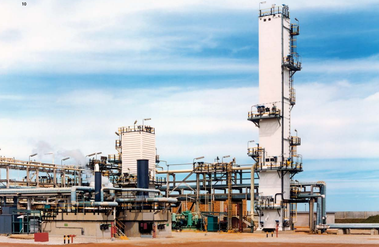
Linde cold boxes in a LNG peak shaving plant
