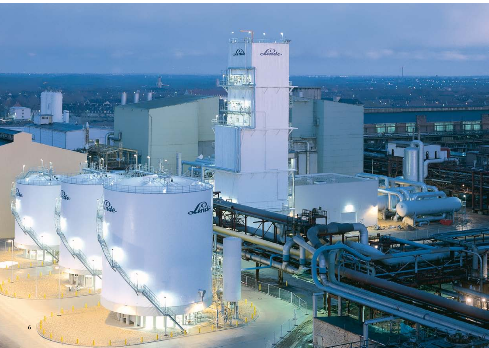
Air separation plant in Leuna, Germany
