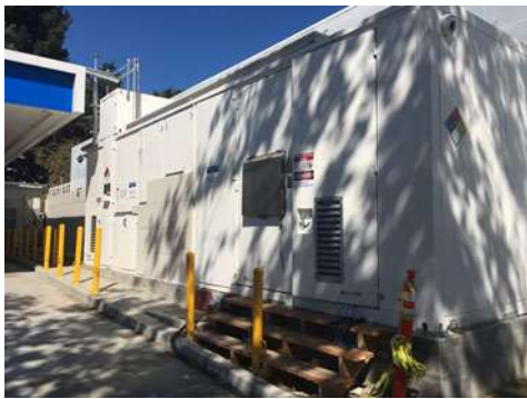
Containerized hydrogen fueling solution including Cryopump CP90 and 800 kg liquid hydrogen tank [Source: Linde]00
