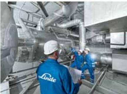
Aluminium plate-fin heat exchanger.
