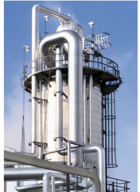
Linde isothermal reactor
