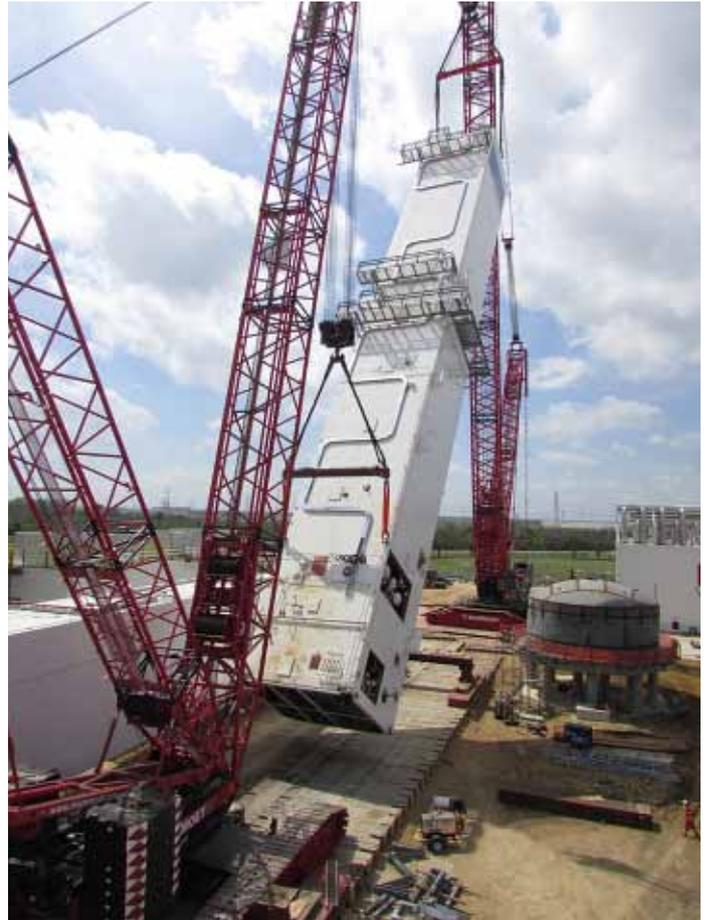
Coldbox erection for a SCALE 60 plant in Texas, USA.
