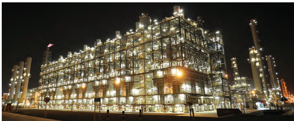
Ethylene furnaces supplied on an EPC basis by Linde Engineering North America Inc. (formerly Selas Fluid Processing)
