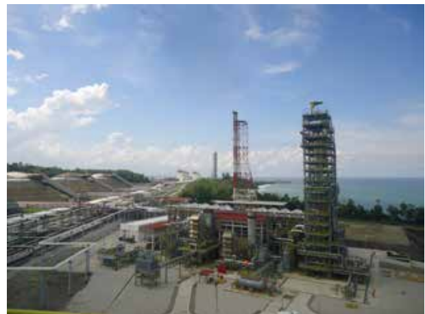
Figure 3. BOG reliquefaction plant in Bintulu, Malaysia.
