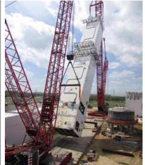
Erecting the coldbox at a NOVON™ plant in Texas, USA.
