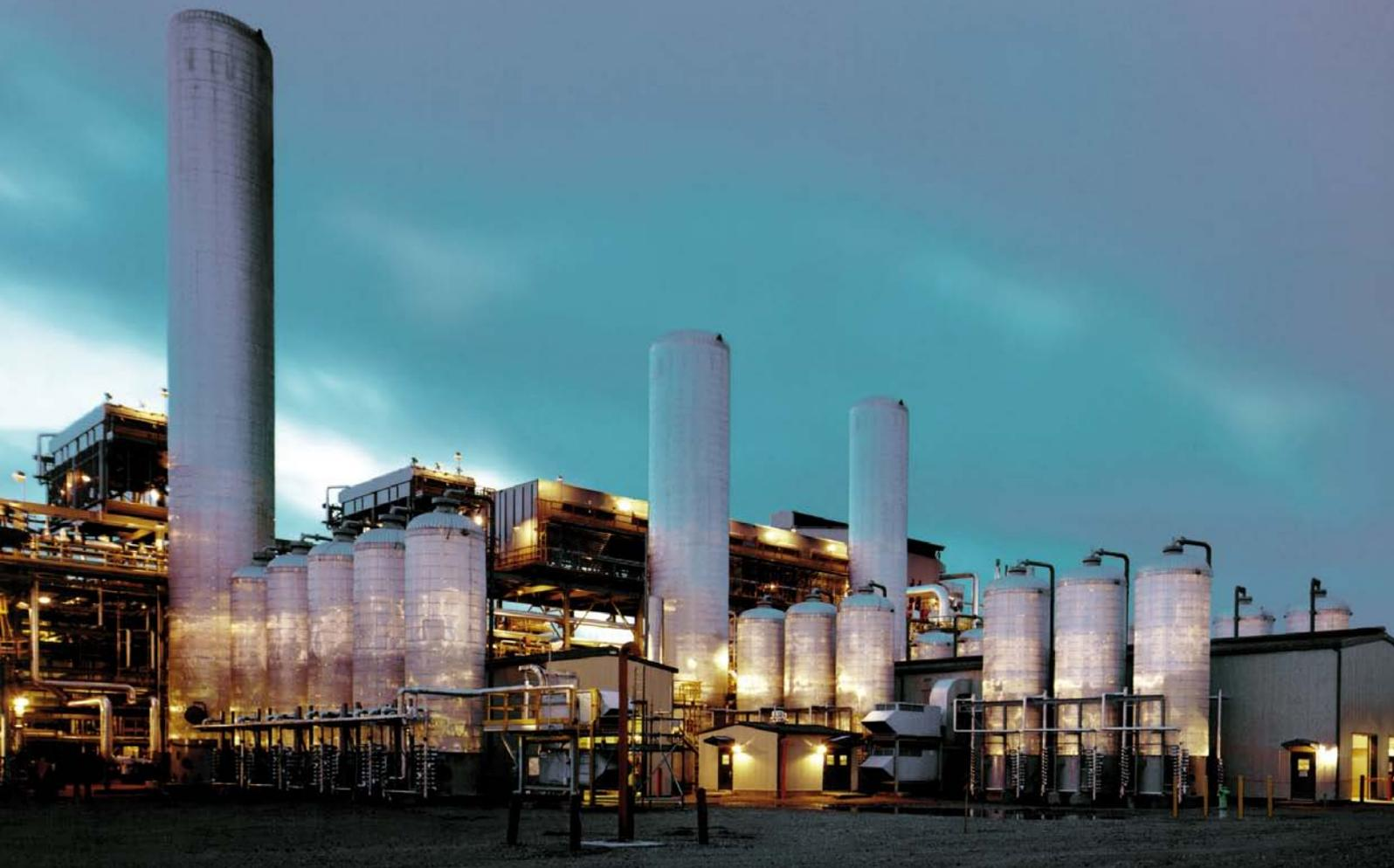
Two pressure swing adsorption units in Canada
